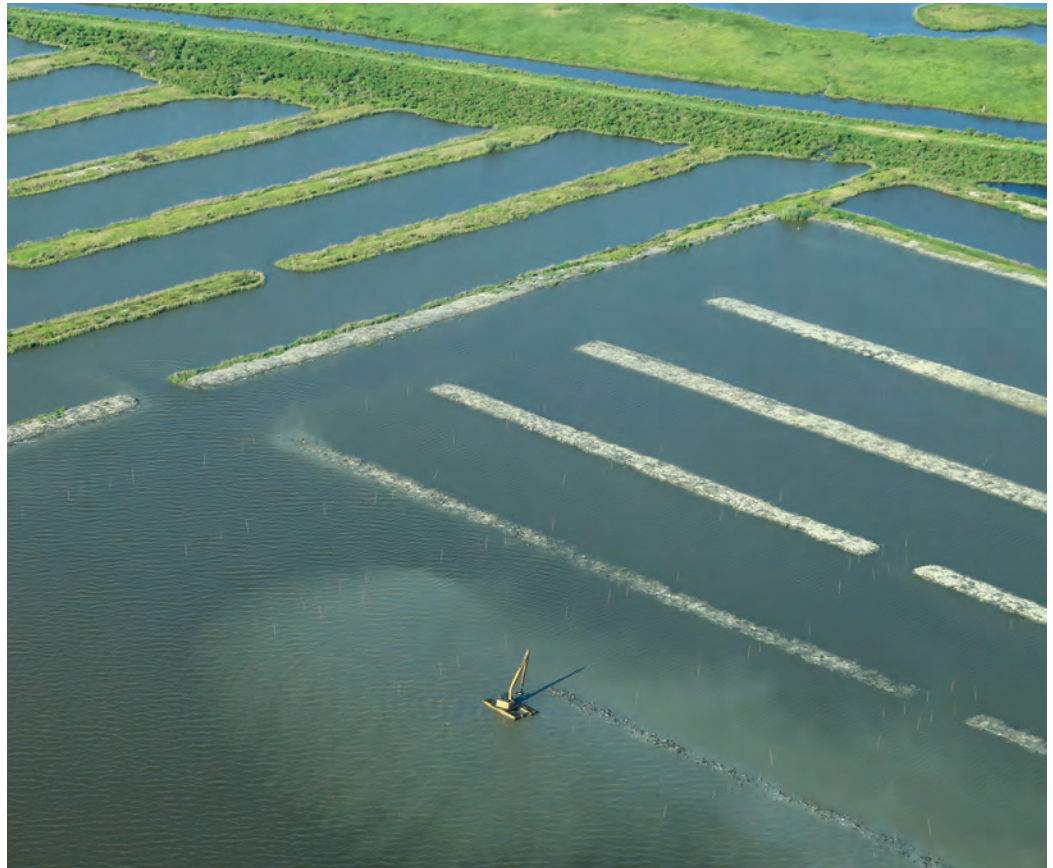
State coastal restoration efforts have included the use of sediment to form terraces intended to slow erosion and ultimately help rebuild fragile marshes.
